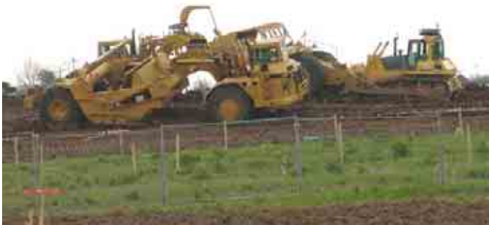
Figure A1.16.2 Site Operation
