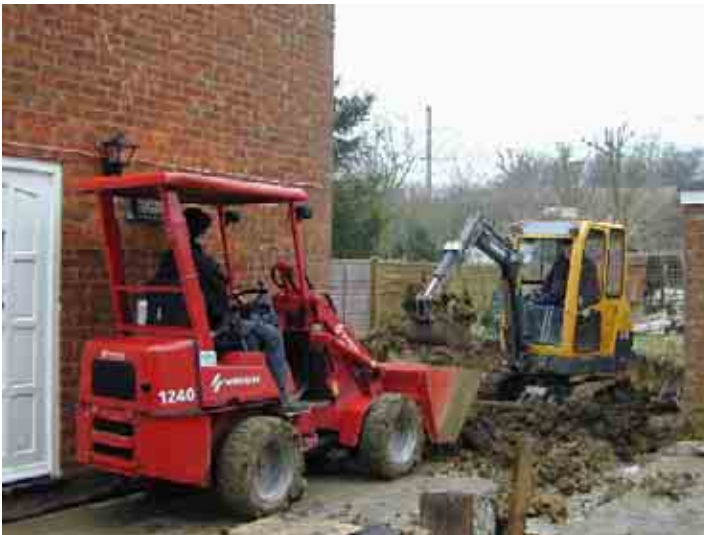
Figure A1.13.1 Volvo EC15B 1.5 tonne compact 360° excavator excavating footings for house extension and patio
