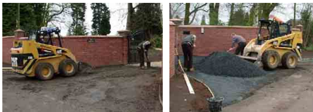
Figure A1.15.1 Site Operation
