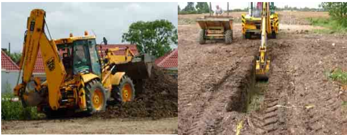
Figure A1.1.1 JCB 4CX Super backhoe loader at work on-site
