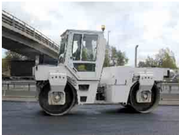
Figure A1.6.1 Bomag BW161 AD2 10-tonne articulated twin-drum vibrating roller compacting freshly-laid hot asphalt on M25
